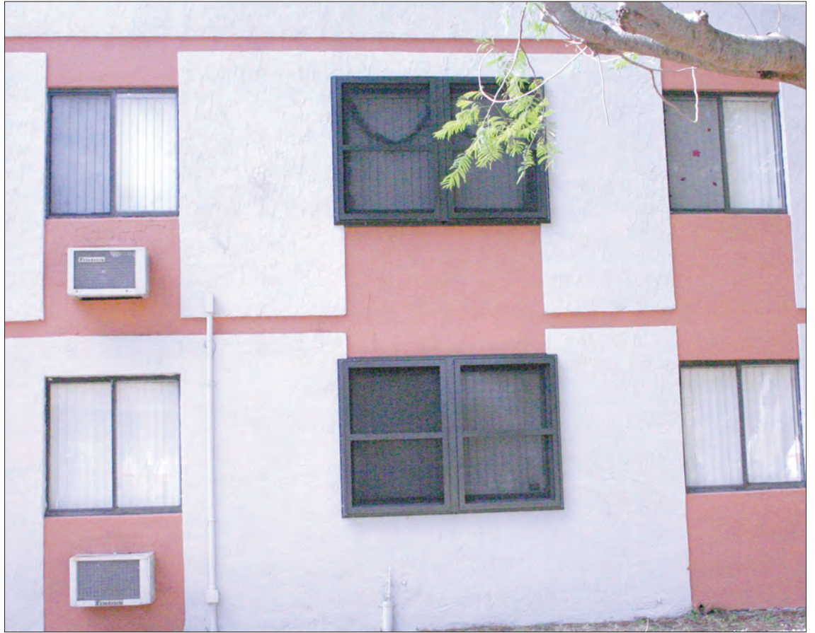
ALL SHUTTERED UP: Hurricane screens installations have begun at UP during the winter break and have made quite a difference in the buildings look. JESSICA MARSHAL/THE BEACON
