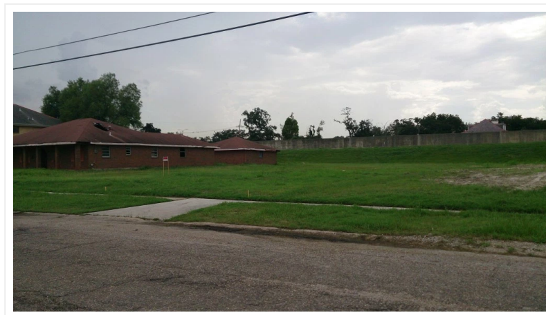
The London Canal Levee, shown here, is where water broke through to flood much of New Orleans in 2005.
