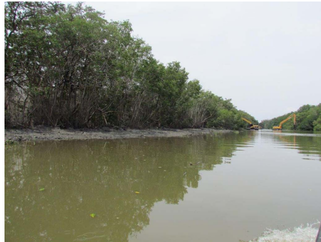
Figure 7. Sediment barriers to hydrologic connectivity. Sediment accumulated along the banks of the artificial channels that act as a barrier to fresh water input into neighboring wetland bodies.
