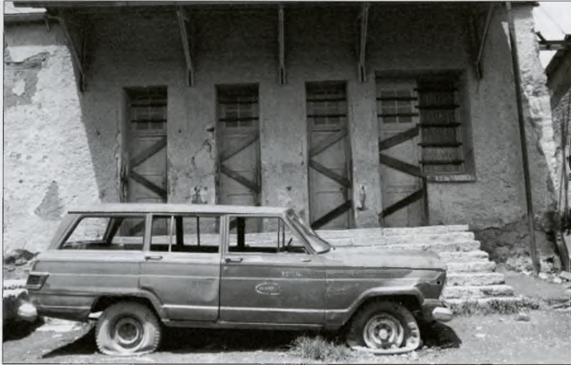
A dilapidated Comibol station wagon parked in front of an abandoned building in the mining town of Catavi. The scene captures the desolation of most mining towns in Bolivia today.
