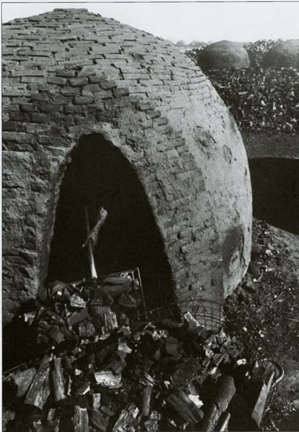
The characteristic round brick ovens used in charcoal production dot an arid landscape in Mato Grosso do Sul.
