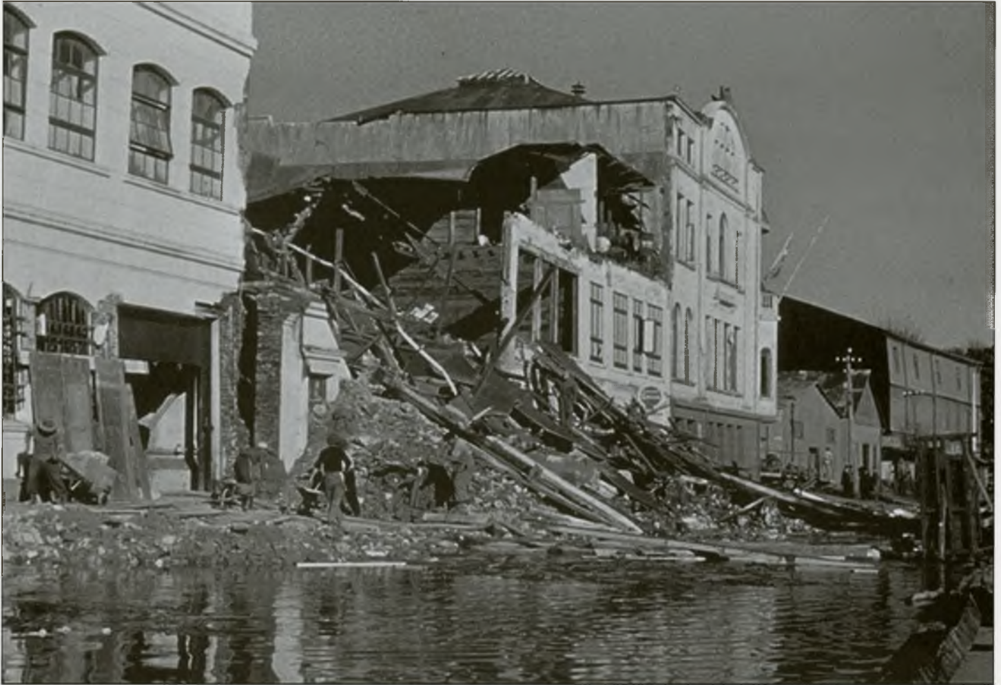
A view of demolished buildings along Costañera Avenue in Valdivia, Chile. This massive earthquake, which convulsed southern Chile in May 1960, registered a magnitude of 8.50. Photo: Steinbrugge Collection, EERC.
