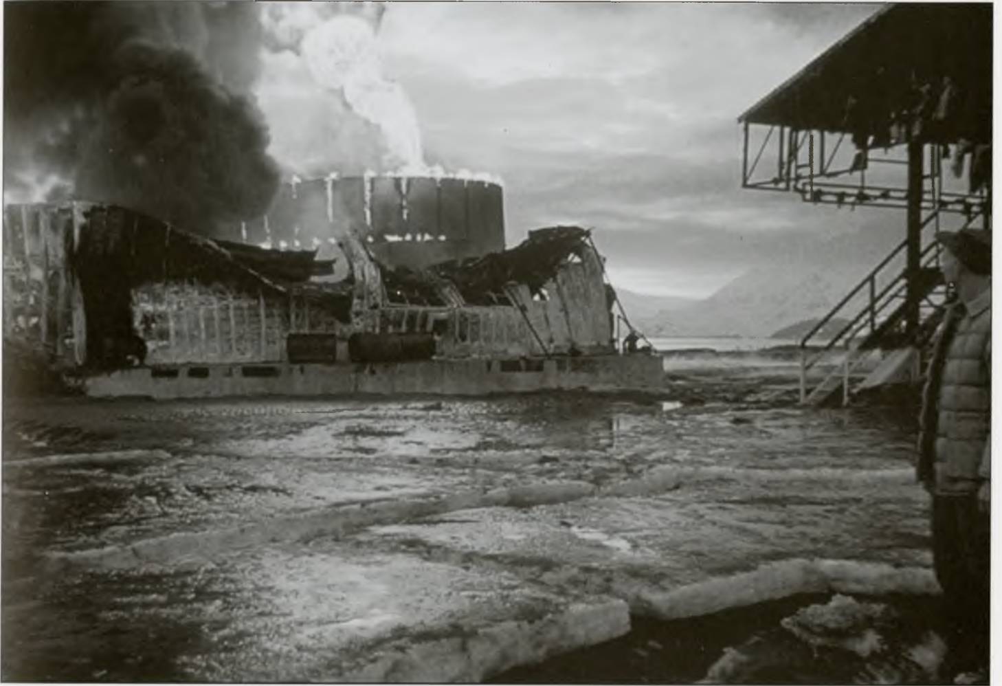
A burning petroleum tank in Valdez, Alaska. This burst of fire was caused by one of the most powerful and longest earthquakes on record—the Anchorage, Alaska, earthquake of March 27, 1964. The tremor measured 8.60 and lasted four minutes. Photo: Steinbrugge Collection, EERC.
