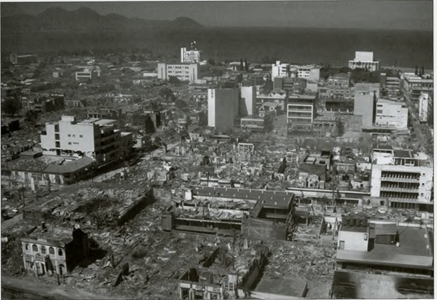
Downtown Managua, Nicaragua, in ruins after the earthquake of December 23, 1972, which measured 6.19. Photo: Steinbrugge Collection, EERC.
