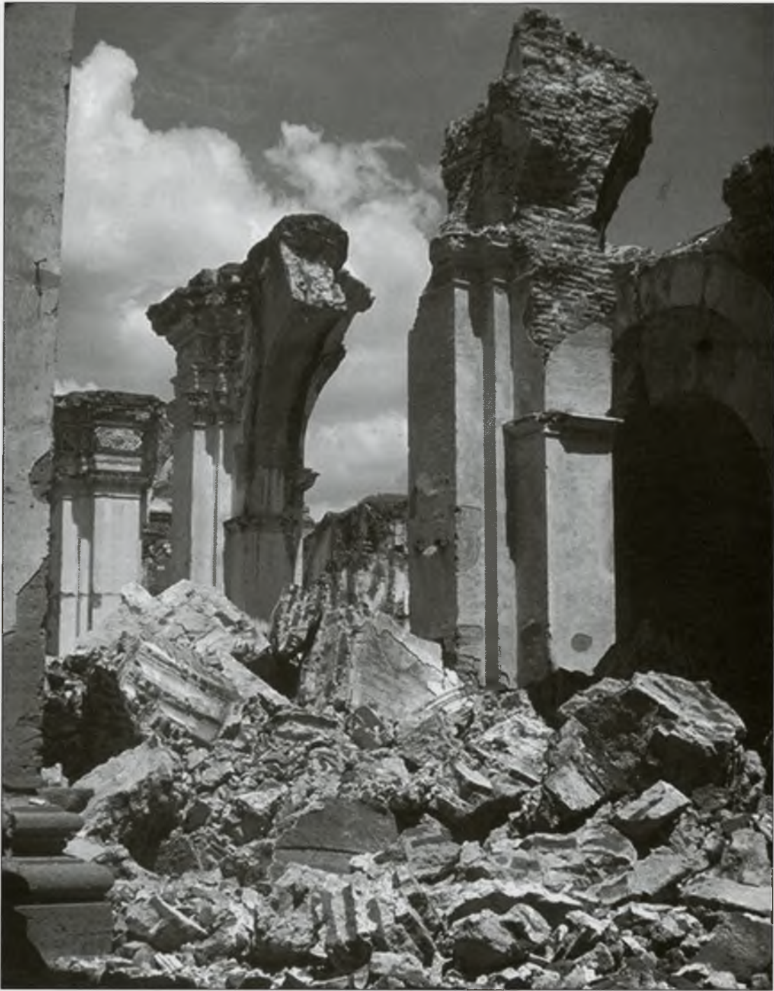
The colonial city of Antigua, Guatemala. Much of Antigua's colonial architecture was devastated by the earthquake of February 4, 1976, which measured 7.50. Photo: Steinbrugge Collection, EERC.
