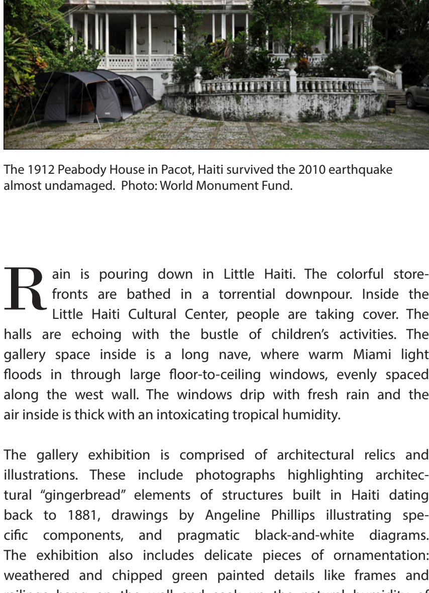
The 1912 Peabody House in Pacot, Haiti survived the 2010 earthquake almost undamaged. Photo: World Monument Fund.
