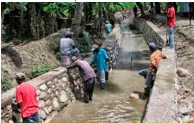
Canal construction Photo: WCDO
