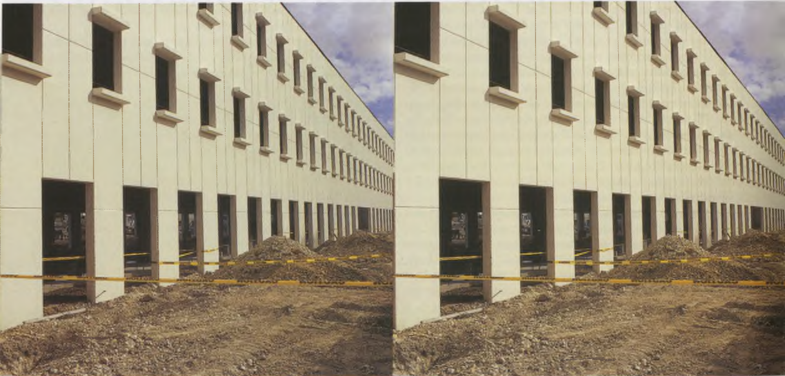
The Bernard Tschumi-designed building for the School of Architecture, seen above, is being constructed with prefabricated exterior walls.
