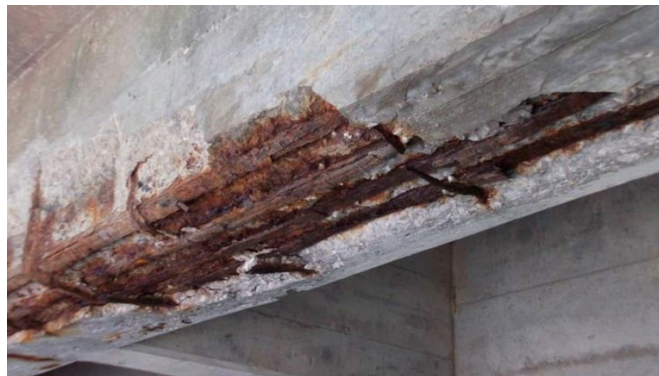
Figure 26 Corrosion in steel reinforcement embedded in concrete substrate (Jung, Jeong, and Lee 2022)
