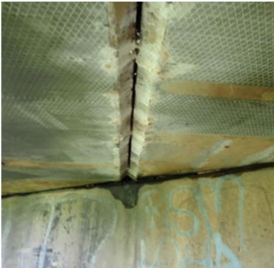
Figure 40 Efflorescence near joints of adjacent box beam girders (Baniya et al. 2022)
