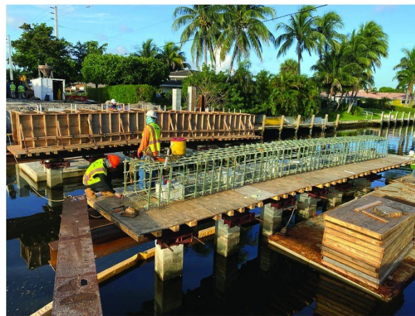
Figure 8 The use of FRP reinforcing bars for piers and bent caps (Broward County, FL, USA) (Ekenel, y Basalo, and Nanni 2021)
