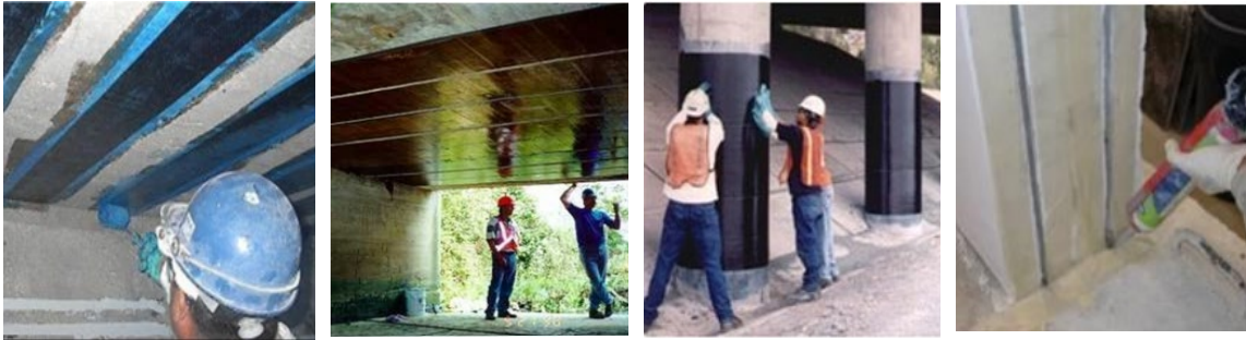
Wet lay-up and, near surface mounted FRP
