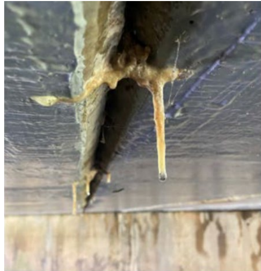
Figure 40 Efflorescence near joints of adjacent box beam girders (Baniya et al. 2022)
