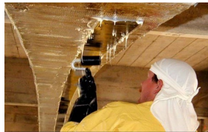
4. Application of pressure onto the applied FRP
