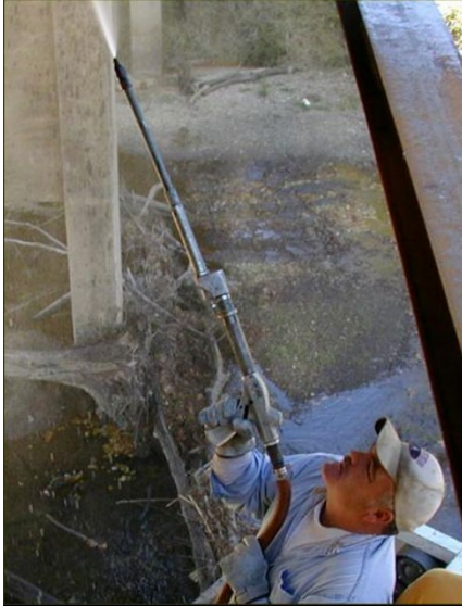
1. Removal of dust, dirt and laitance from the substrate (Hydroblasting)
