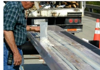
2. Application of resin on FRP and substrate
