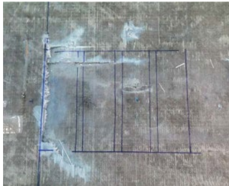
Figure 13 Discoloration (Telang et al. 2006)
