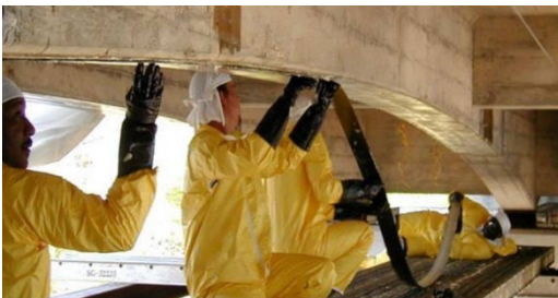
3. Application of FRP on substrate
